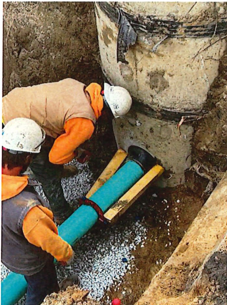
Figure 7: New force main connection to manhole
