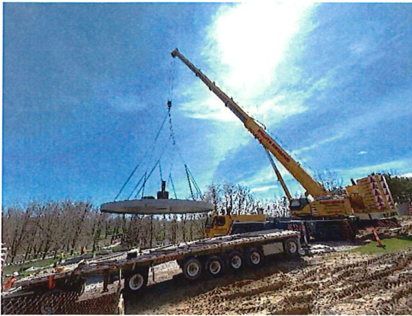
Figure 1: Digester Cover Installation
