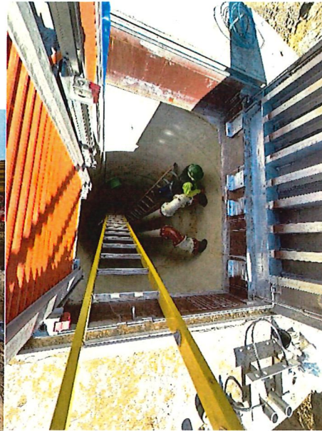
Figure 6: Relocated Lift Station #8 Equipment
