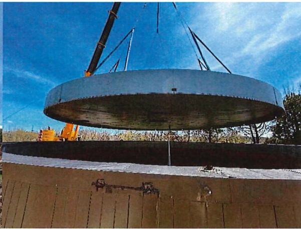
Figure 2: Digester Cover Installation
