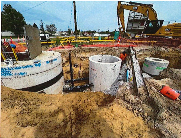
Figure 5: Relocated Lift Station #8 Structures Installed
